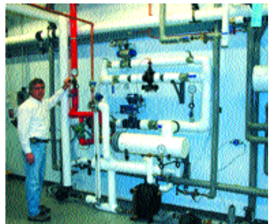
Training Centre, Allentown, USA.
